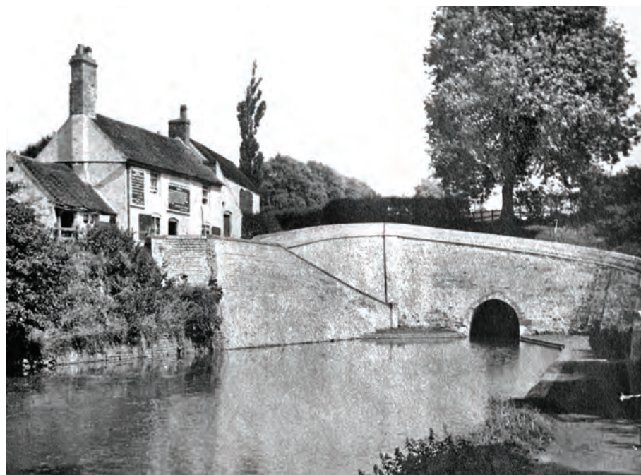
The west portal of Lapal Tunnel at Halesowen. The toll house is seen on the left. Tunnel charges are displayed on a board outside.
